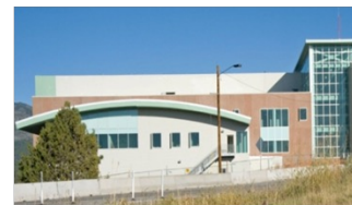
CMR Replacement (CMRR) Building
