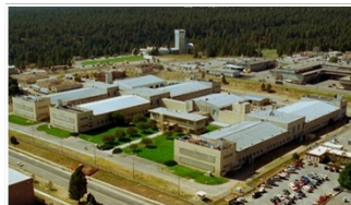
Chemistry and Metallurgy Research (CMR) Bldg.
